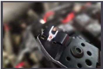
Strip the cable and crimp the supplied cable forks onto the cable.
